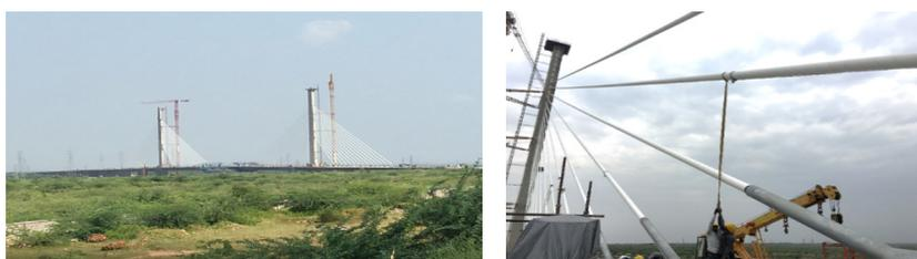
Figure 9: Construction of Kota Chambal Bridge (left), with monitoring of many variables including stay cable vibrations (the picture on the right shows forced vibration of a stay cable with an accelerometer)
