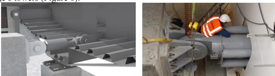
Figure 6: An STU at each tower of the Hålogaland Bridge controls superstructure movements – design representation (left) and during installation (right)
