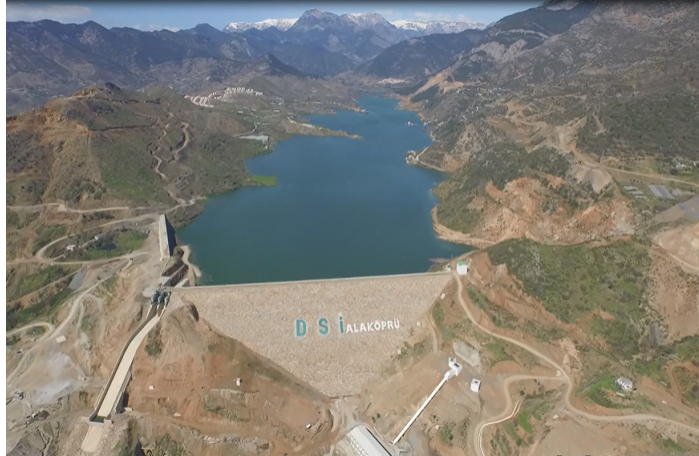
Figure 3: Alaköprü Dam and reservoir
