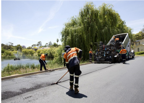
Figure 1 : Road developed from plastic bags and glass bottles in Australia (Onkaparinganow, 2018; Department of the Environment and Energy, Australian Government, 2019)
