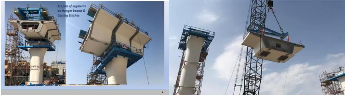
**Fig. 5:** Precast Concrete Segment Installation for Junction B6 bridge
