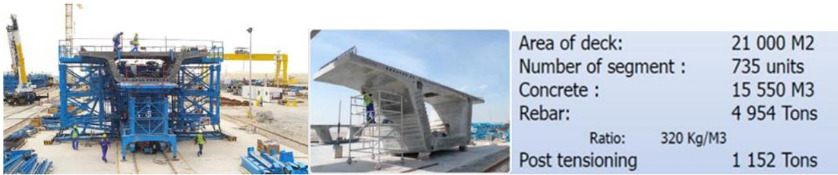
**Fig. 4:** Precast Concrete Segment Fabrication in VSL Yard 50 kms. south of Doha
