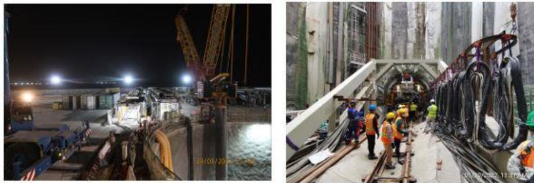
**Fig. 7: TBM Umbilical site setup**
