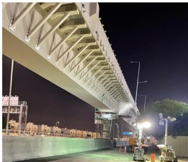
**Fig. 12:** The Completed Deck Extension (site photo)
