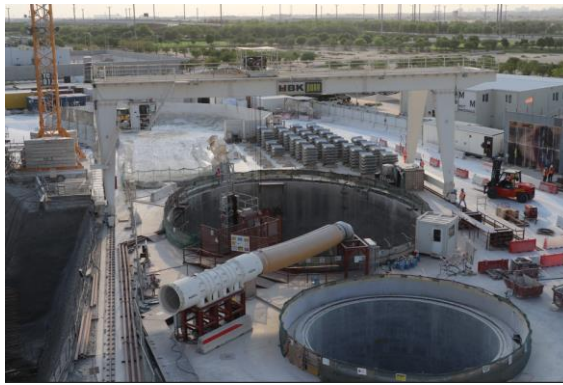
Fig. 9: Photo of the logistics and drop shafts during TBM operations
