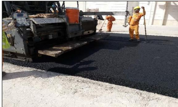
**Fig. 3:** Paving Operations of Asphalt Mix with 15% RAP
