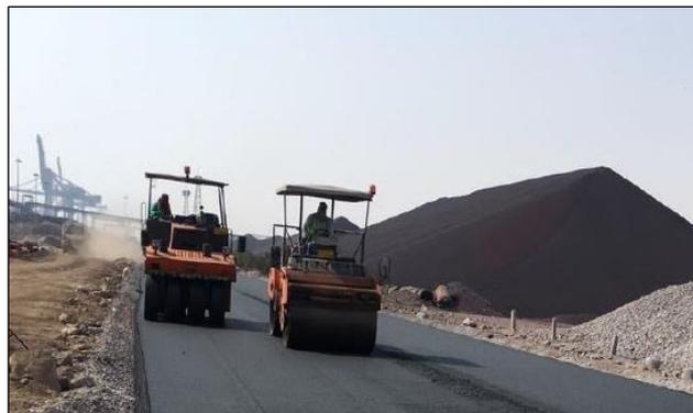
**Fig. 4:** Paving Operations of Asphalt Mix with 20% steel slag
