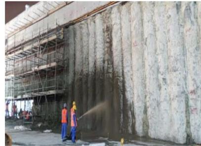
Application of Shotcrete at inner face of piles
