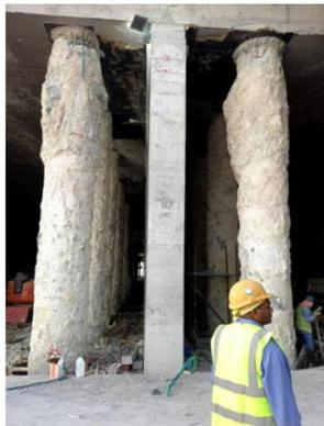
Casting Central wall in between temporary piles
