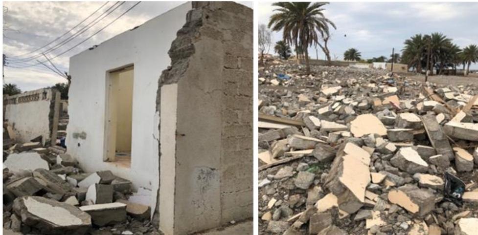
**Fig. 1:** Examples of Demolition Waste from Al-Masnaah- Al Batanah Region – Oman
