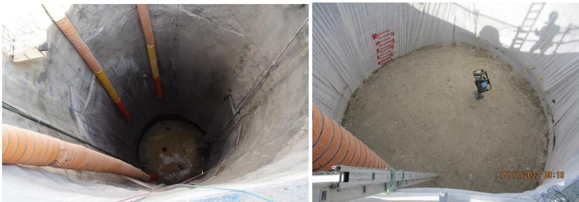
**Fig. 1:** Temporary shafts on the WWDNB project used for micro tunneling and manhole installation (left side) and ongoing conventional backfilling works (right side)
