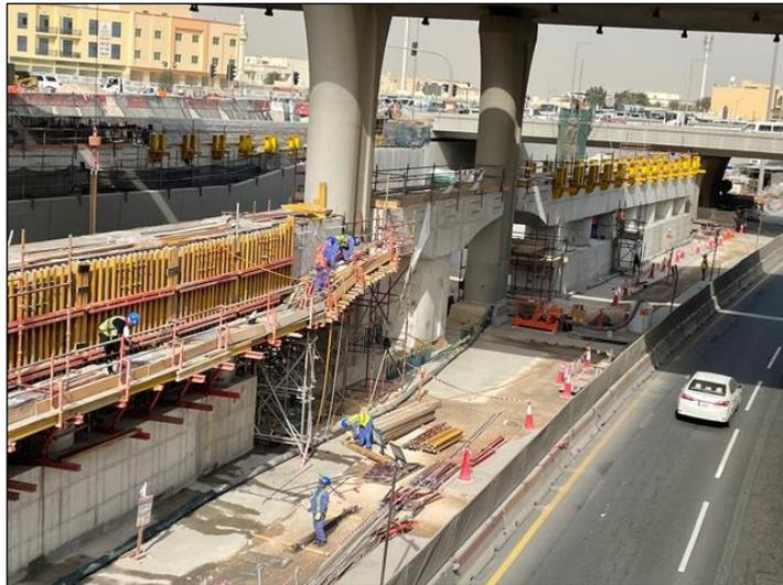
**Fig. 9:** – Median Piers during construction
