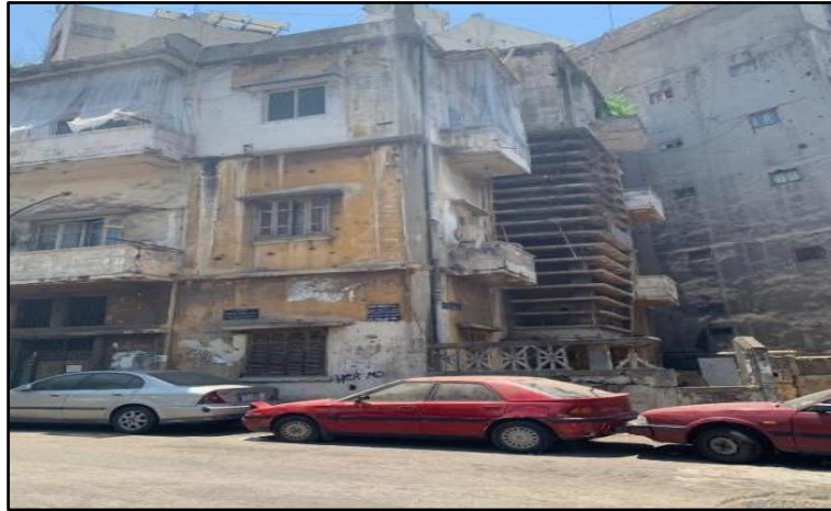
Fig. 42: Photo showing Al-Tamlis building before intervention
