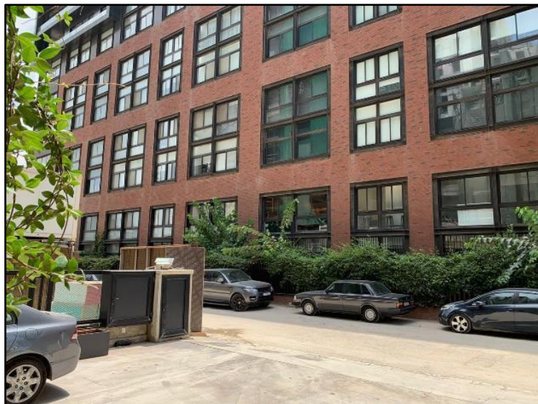
Fig. 30: Factory 4376 Building Before intervention
